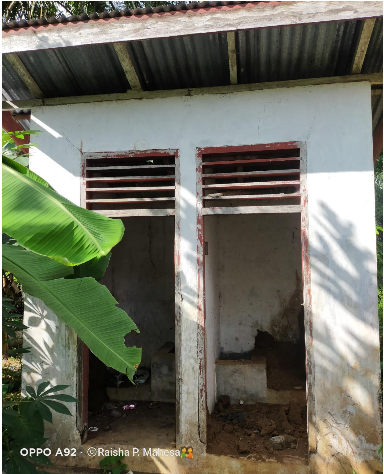
Photo keadaan wc
